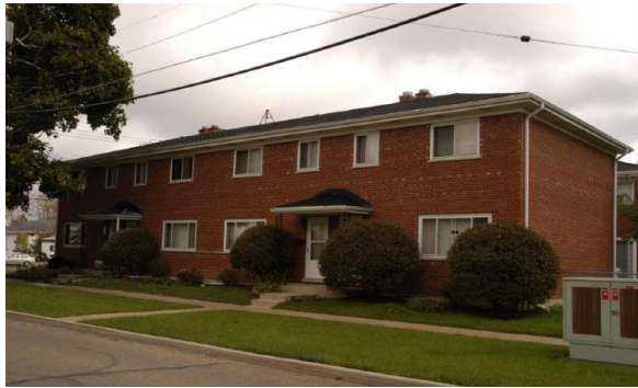
All Separate utilities including Water/Sewer
